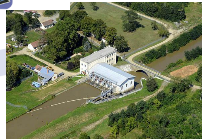
Ikervár Hydroelectric Plant (1896): Built earlier on the Rába River, it stands as Hungary's first hydroelectric power plant utilizing water energy for electricity.
